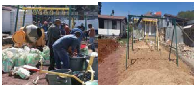
Fixation of outdoor children playing materials at Asco SC rehabilitation center
